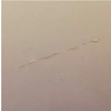
Initial situation after the curing time
